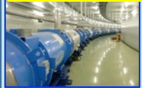
Superconducting D-Q combined function magnet
